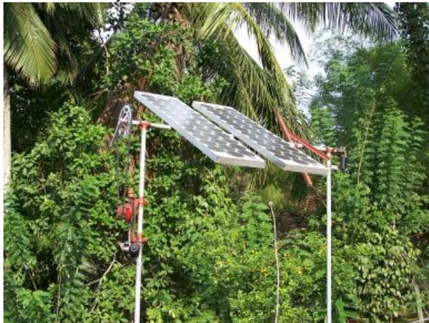
But it was very clear that when the panels are placed directly facing the sun, the efficiency becomes considerably higher. Therefore, I have decided to mount the panels in a mechanical arrangement, whereby I can
